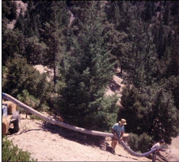
Figure 6-18. Using Straw Blower to Apply Mulch
