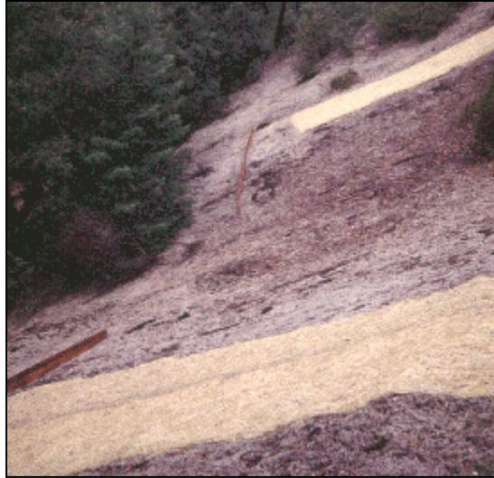
Figure 6-16. Erosion Blankets
