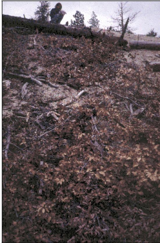
Figure 6-9. Slash Spread on a Sheet and Rill Slope
