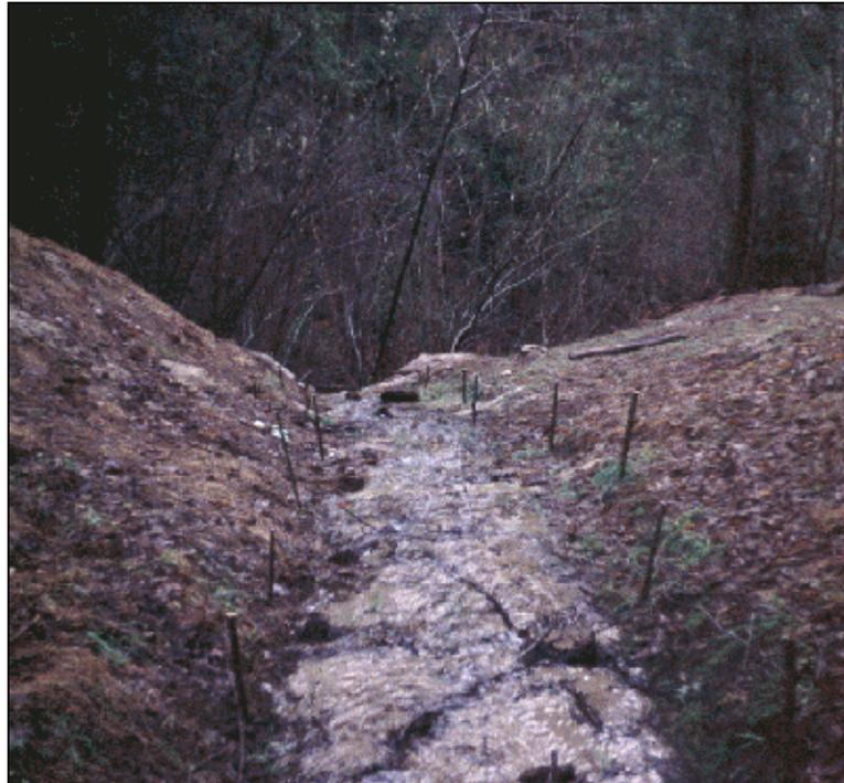
Figure 6-7. Willow Stakes Installed Along an Excavated Channel
