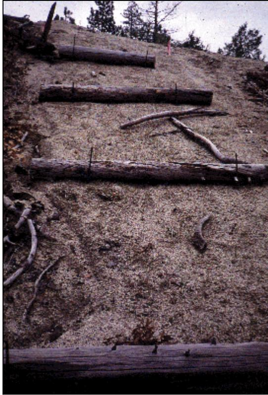
Figure 6-15. Cross Slope with Logs
