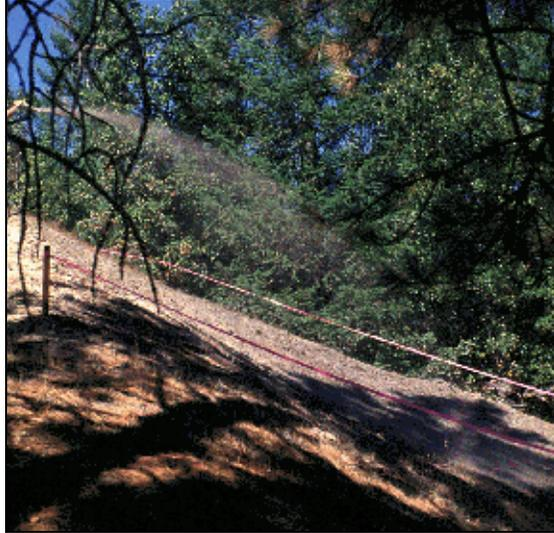
Figure 6-17. Lime-Based Tackifier Being Applied
