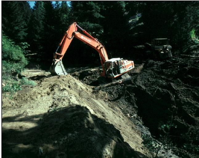
Figure 3-4. Heavy Equipment Removing a Road Crossing.
