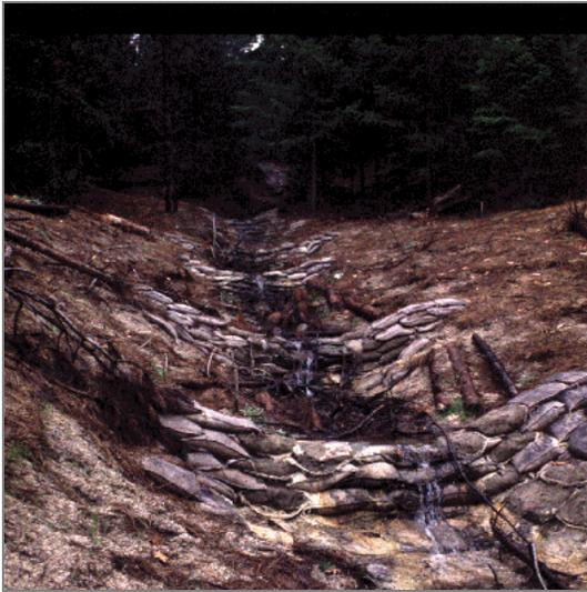
Figure 5-10. Soil/Cement Checkdam
