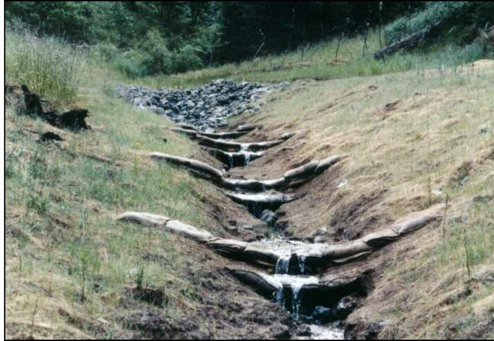
Figure 3-2. Soil/Cement Grade Stabilization Structure.
